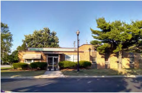
Department of Public Works Building
