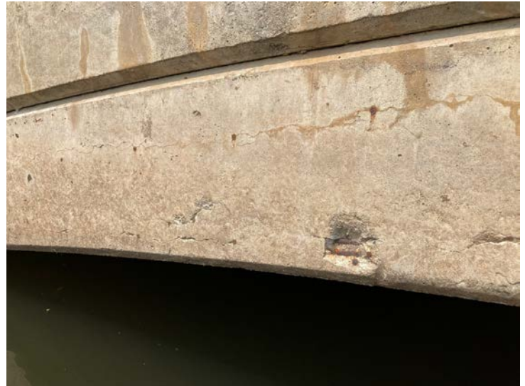
Document Name: IMG_4642.JPG Category: Culvert Span Number: Comments: STS in fascia
