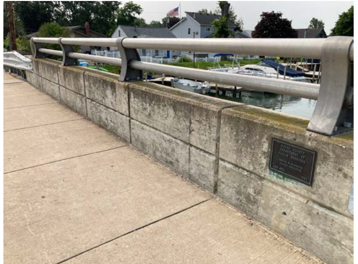
Document Name: IMG_4538.JPG Category: Railing Span Number: Comments: South rail
