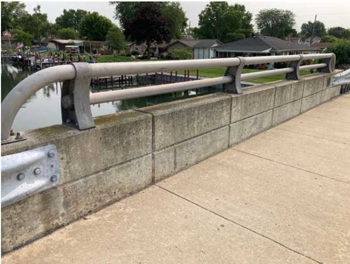
Document Name: IMG_4541.JPG Category: Railing Span Number: Comments: North rail
