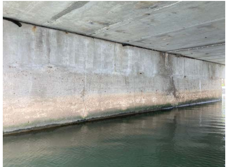
Document Name: IMG_4545.JPG Category: Substructure Span Number: Comments: West abutment
