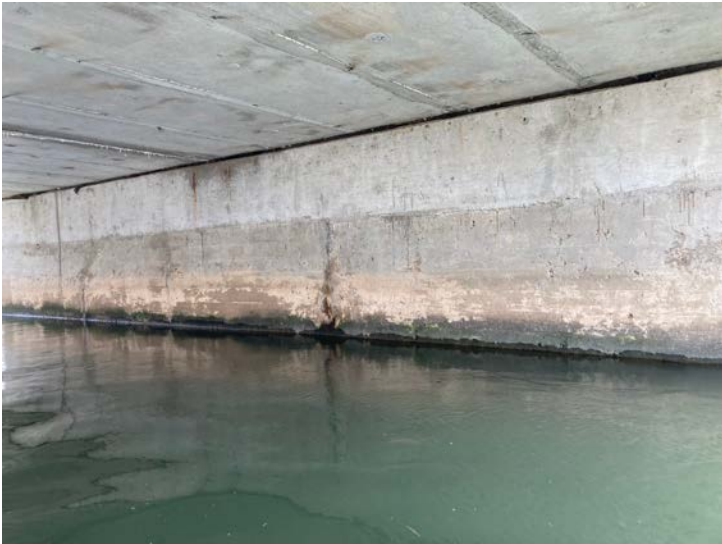
Document Name: IMG_4546.JPG Category: Substructure Span Number: Comments: East abutment
