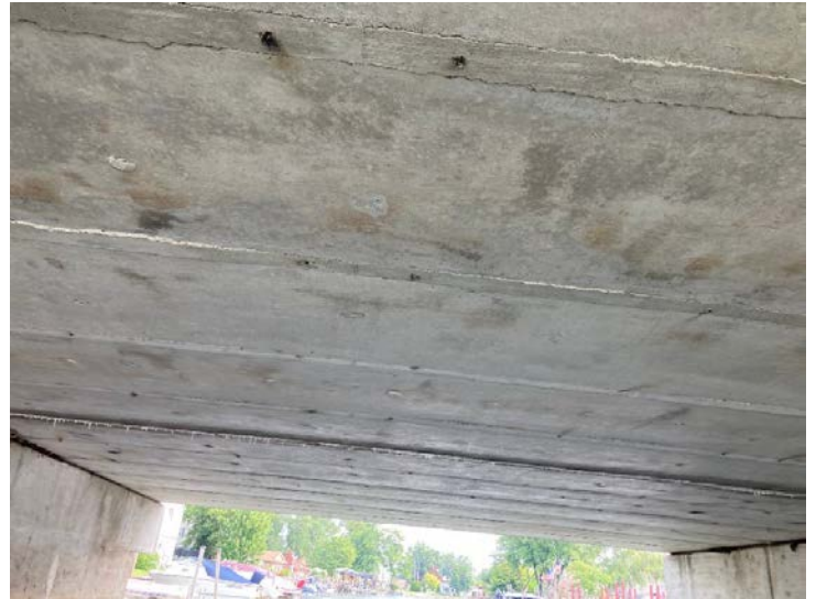
Document Name: IMG_4547.JPG Category: Superstructure Span Number: Comments: Beams
