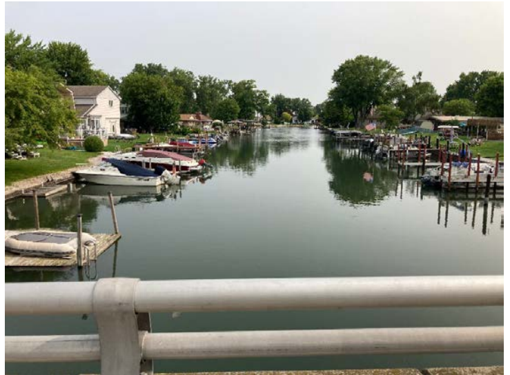
Document Name: IMG_4542.JPG Category: Channel Span Number: Comments: North channel
