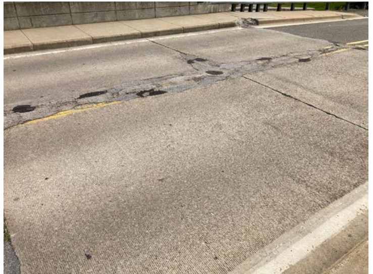
Document Name: IMG_4534.JPG Category: Deck Span Number: Comments: Deck surface
