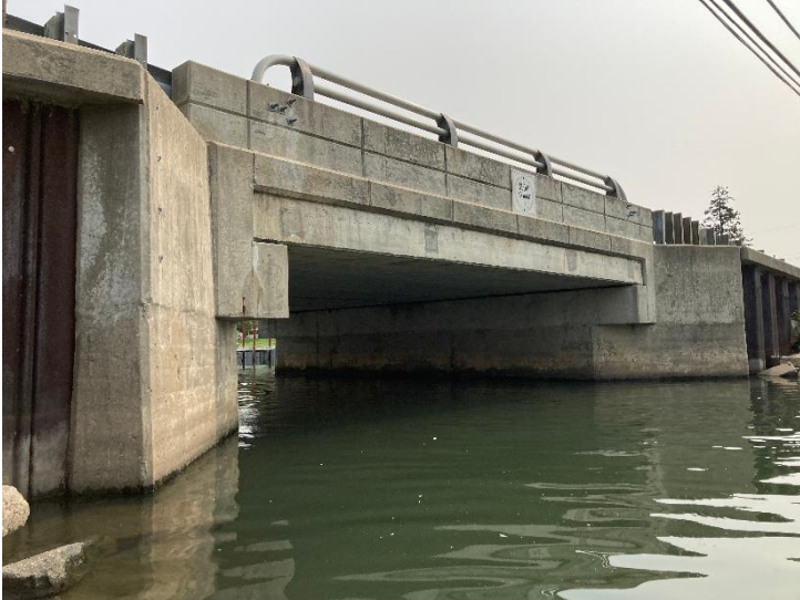
Document Name: IMG_4544.JPG Category: Elevation Span Number: Comments: South elevation
