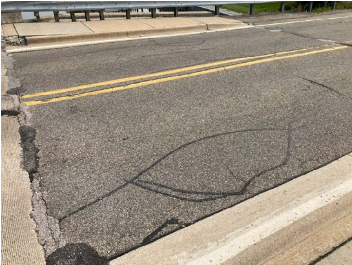
Document Name: IMG_4536.JPG Category: Approach Span Number: Comments: East approach
