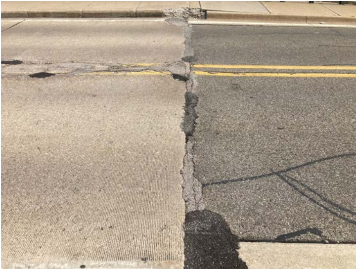
Document Name: IMG_4535.JPG Category: Joints Span Number: Comments: East reference line
