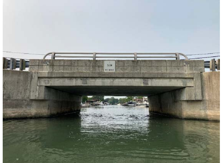
Document Name: IMG_4550.JPG Category: Elevation Span Number: Comments: North elevation
