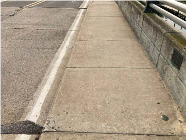
Document Name: IMG_4537.JPG Category: Deck Span Number: Comments: South sidewalk
