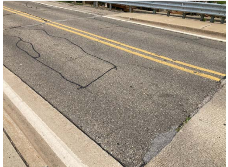
Document Name: IMG_4532.JPG Category: Approach Span Number: Comments: West approach
