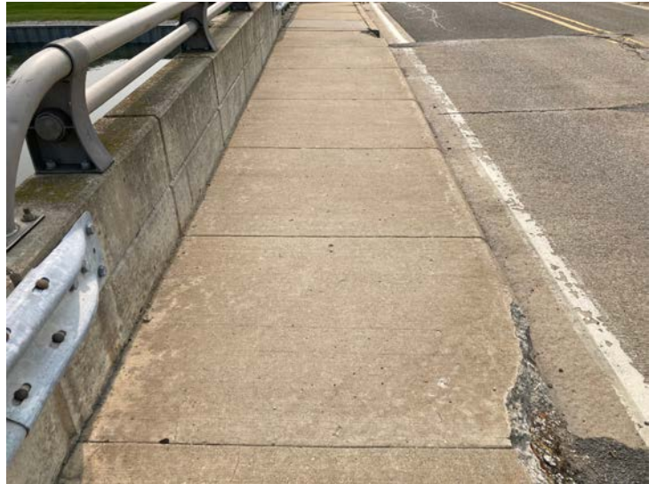
Document Name: IMG_4540.JPG Category: Deck Span Number: Comments: North sidewalk
