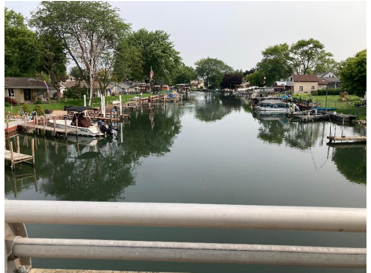
Document Name: IMG_4563.JPG Category: Channel Span Number: Comments: North channel
