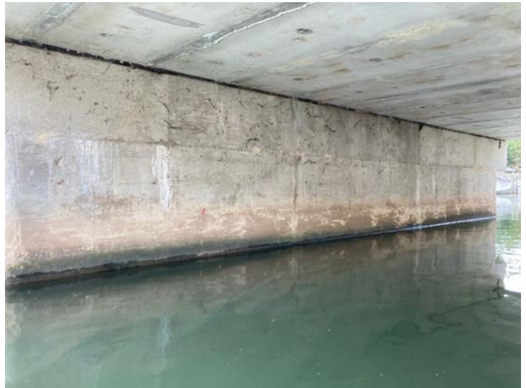
Document Name: IMG_4566.JPG Category: Substructure Span Number: Comments: East abutment
