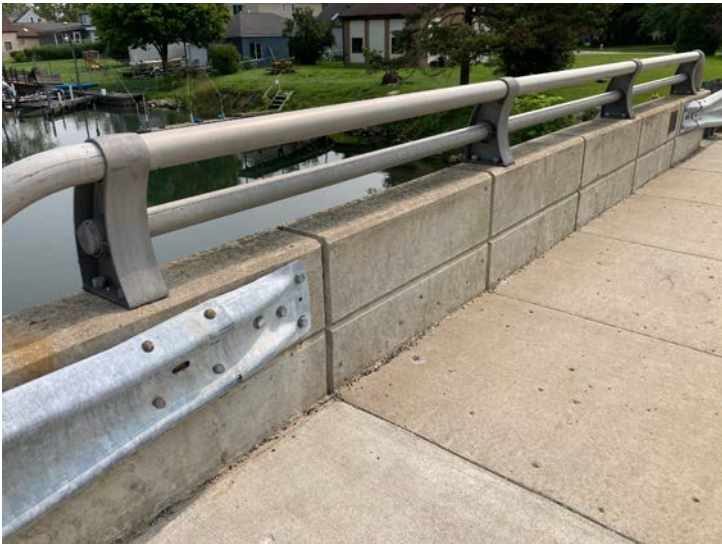
Document Name: IMG_4562.JPG Category: Railing Span Number: Comments: North rail
