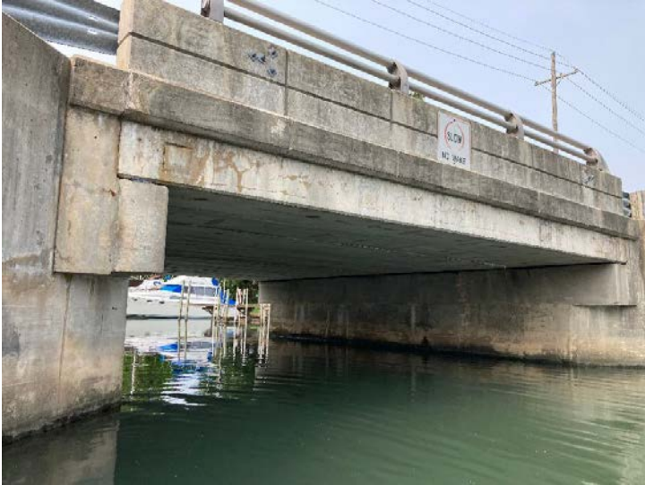
Document Name: IMG_4564.JPG Category: Elevation Span Number: Comments: North elevation
