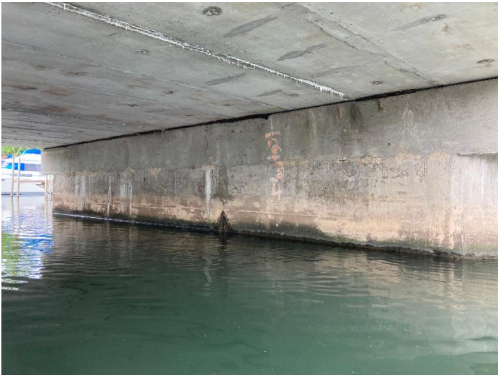
Document Name: IMG_4565.JPG Category: Substructure Span Number: Comments: West abutment
