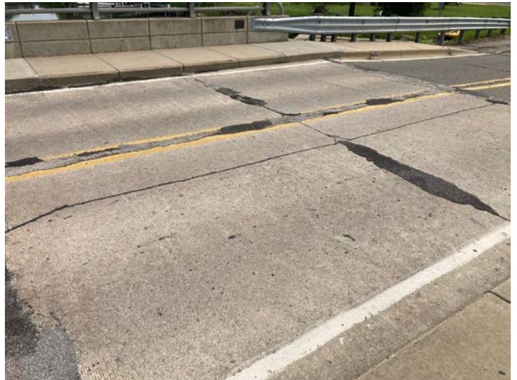
Document Name: IMG_4555.JPG Category: Deck Span Number: Comments: Deck surface
