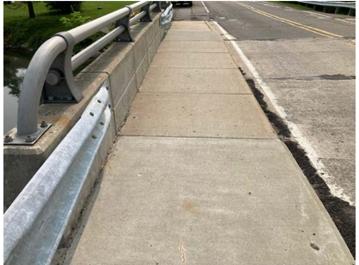
Document Name: IMG_4561.JPG Category: Deck Span Number: Comments: North sidewalk
