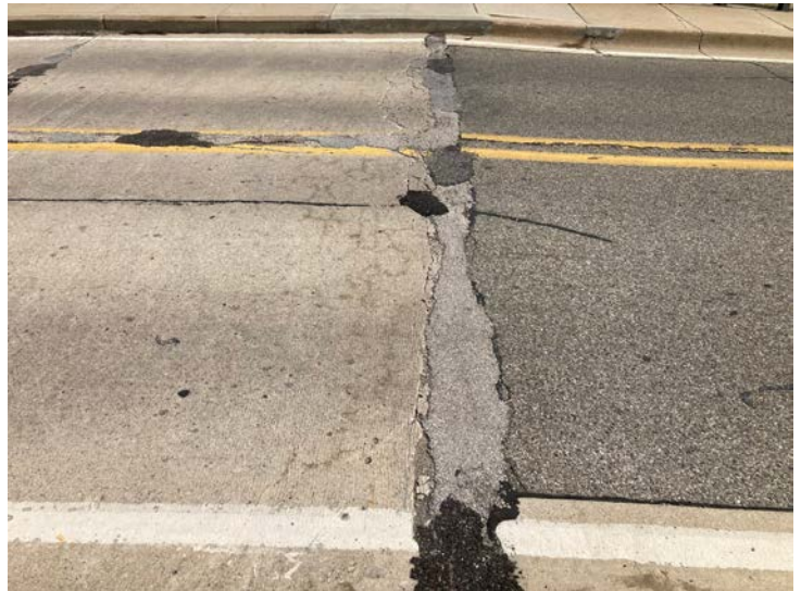
Document Name: IMG_4556.JPG Category: Joints Span Number: Comments: East reference line
