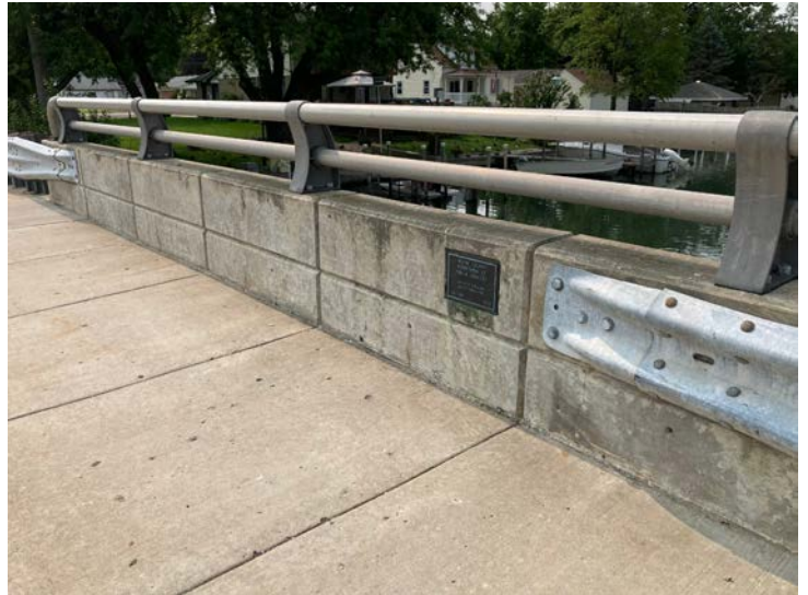
Document Name: IMG_4559.JPG Category: Railing Span Number: Comments: South rail
