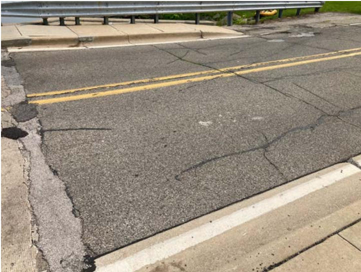
Document Name: IMG_4557.JPG Category: Approach Span Number: Comments: East approach
