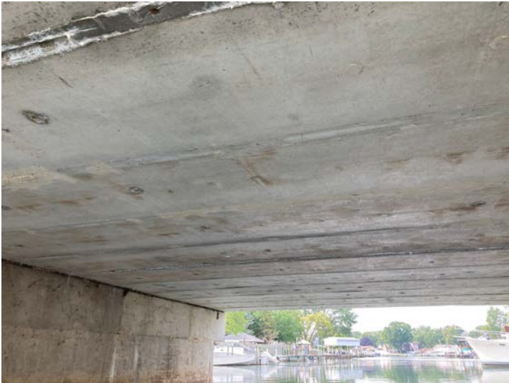
Document Name: IMG_4567.JPG Category: Superstructure Span Number: Comments: Beams
