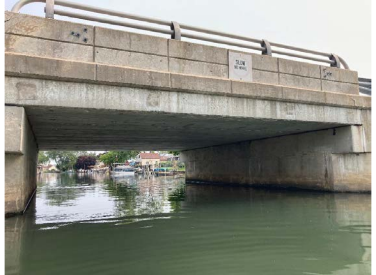
Document Name: IMG_4569.JPG Category: Elevation Span Number: Comments: South elevation
