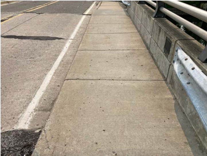
Document Name: IMG_4558.JPG Category: Deck Span Number: Comments: South sidewalk
