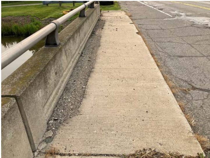
Document Name: IMG_4500.JPG Category: Deck Span Number: Comments: North sidewalk
