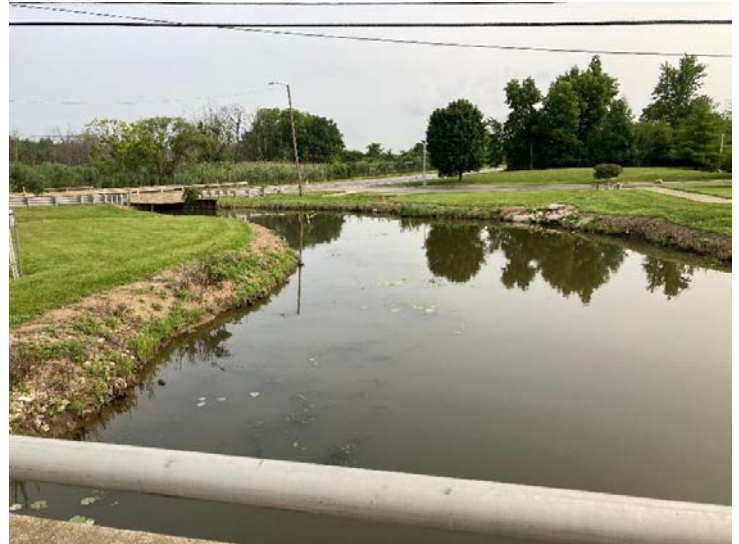
Document Name: IMG_4502.JPG Category: Channel Span Number: Comments: North channel
