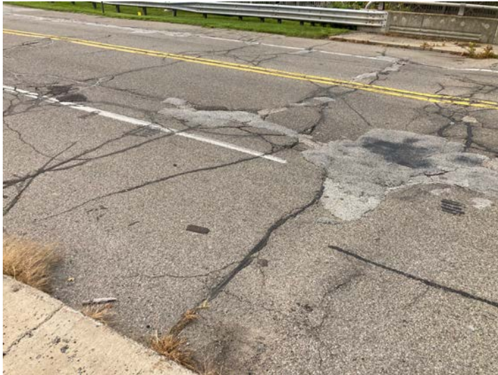
Document Name: IMG_4495.JPG Category: Approach Span Number: Comments: East approach
