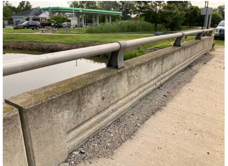
Document Name: IMG_4501.JPG Category: Railing Span Number: Comments: North rail
