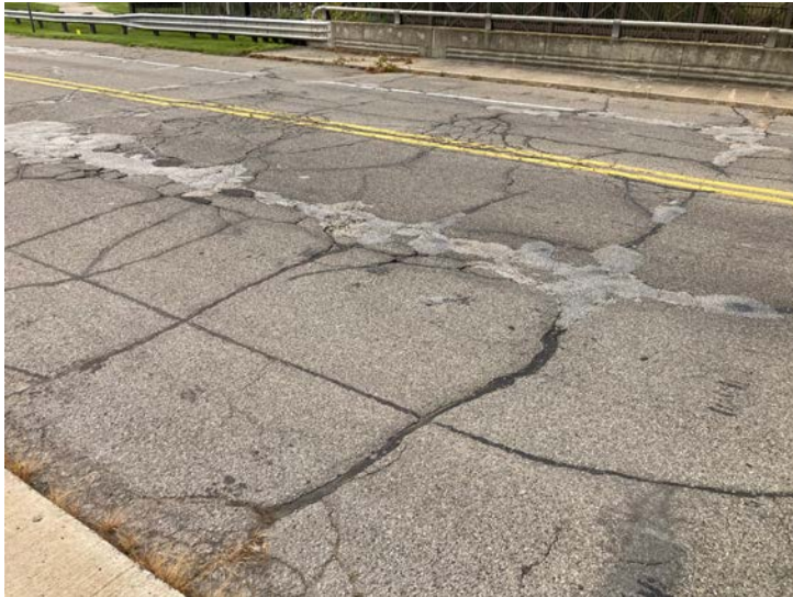
Document Name: IMG_4494.JPG Category: Deck Span Number: Comments: HMA surface
