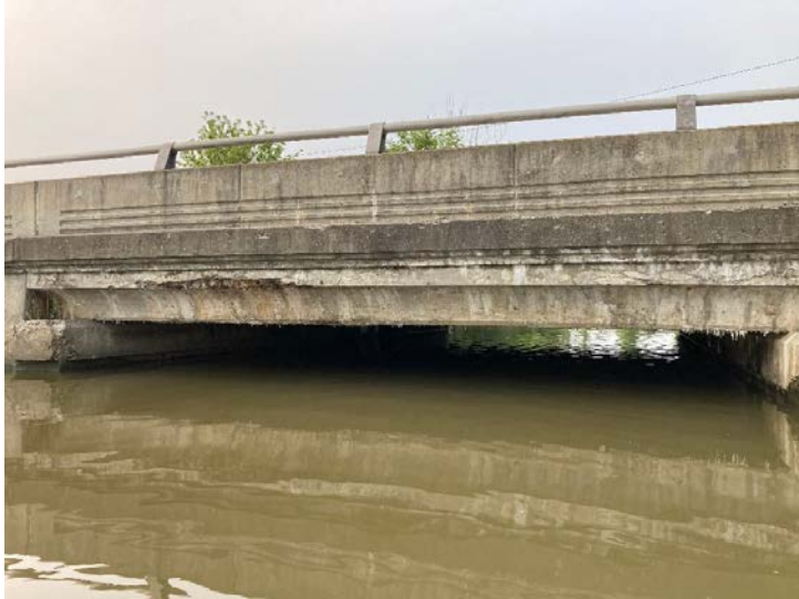
Document Name: IMG_4503.JPG Category: Elevation Span Number: Comments: North elevation
