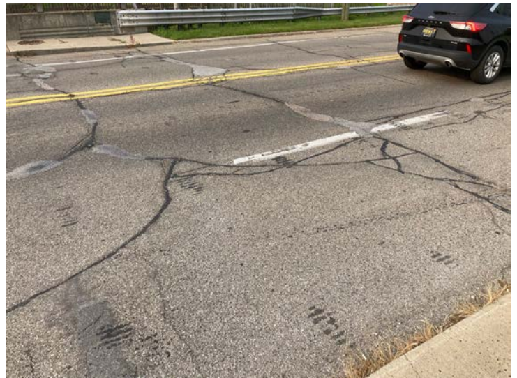
Document Name: IMG_4493.JPG Category: Approach Span Number: Comments: West approach
