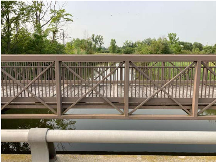
Document Name: IMG_4498.JPG Category: Channel Span Number: Comments: South channel
