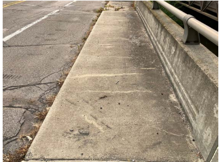
Document Name: IMG_4496.JPG Category: Deck Span Number: Comments: South sidewalk
