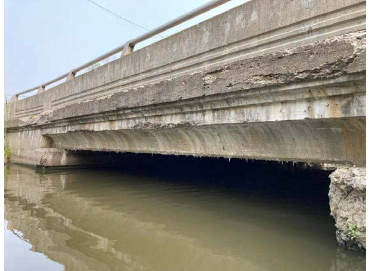
Document Name: IMG_4509.JPG Category: Elevation Span Number: Comments: South elevation
