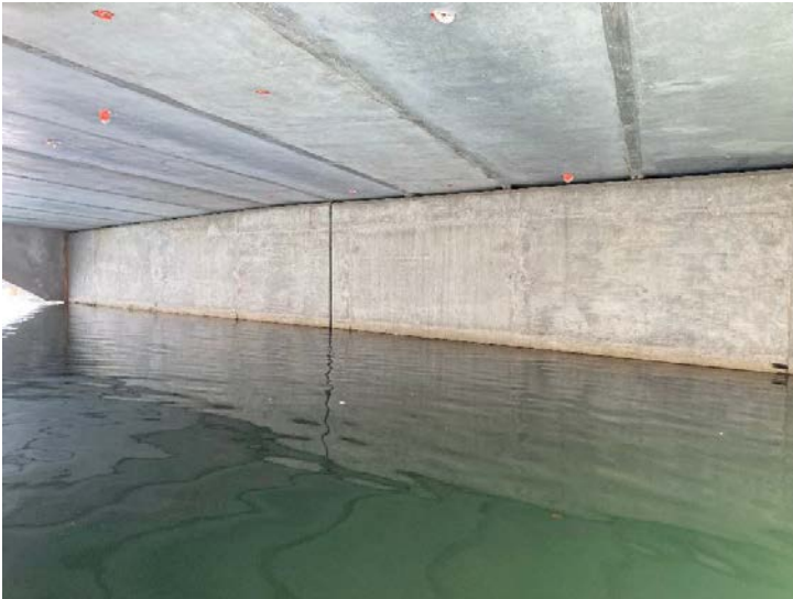
Document Name: IMG_4527.JPG Category: Substructure Span Number: Comments: East abutment
