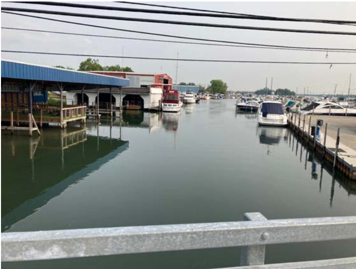
Document Name: IMG_4522.JPG Category: Channel Span Number: Comments: North channel
