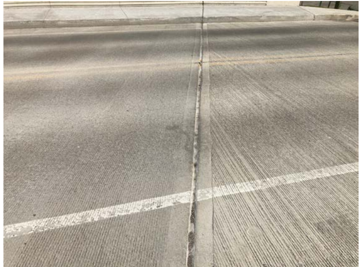
Document Name: IMG_4515.JPG Category: Joints Span Number: Comments: East reference line
