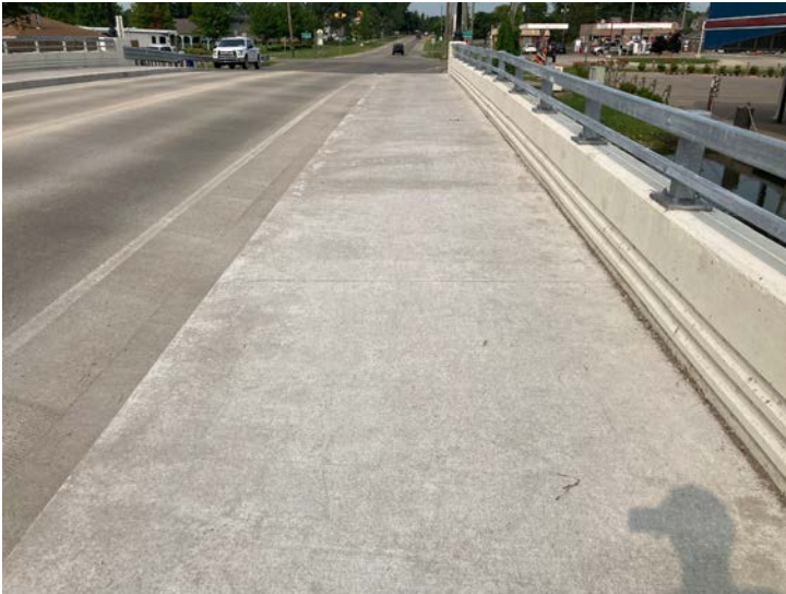
Document Name: IMG_4520.JPG Category: Deck Span Number: Comments: North sidewalk
