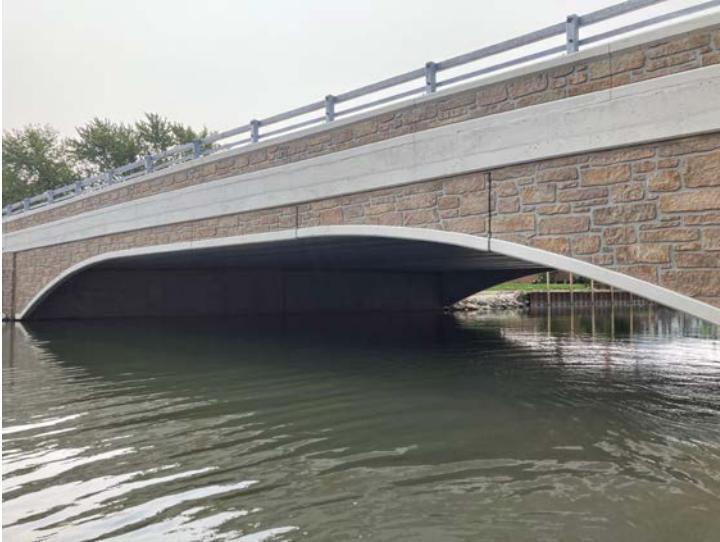
Document Name: IMG_4525.JPG Category: Elevation Span Number: Comments: North elevation
