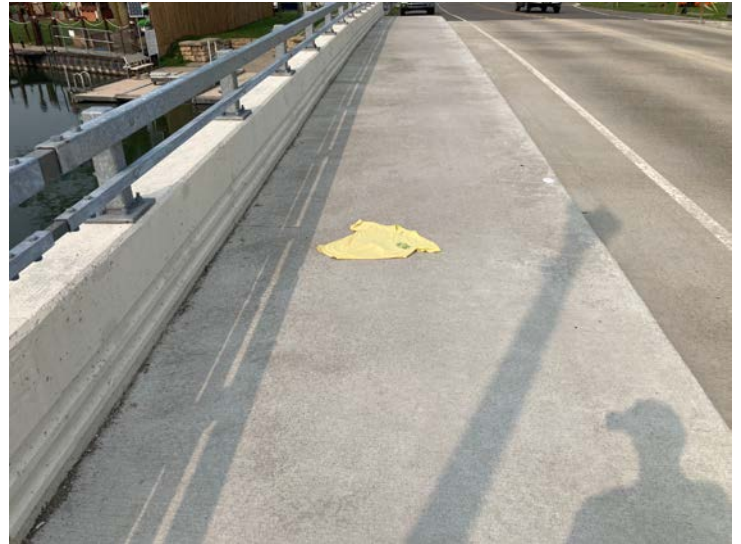
Document Name: IMG_4517.JPG Category: Deck Span Number: Comments: South sidewalk
