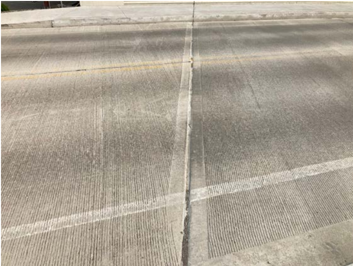
Document Name: IMG_4513.JPG Category: Joints Span Number: Comments: West reference line
