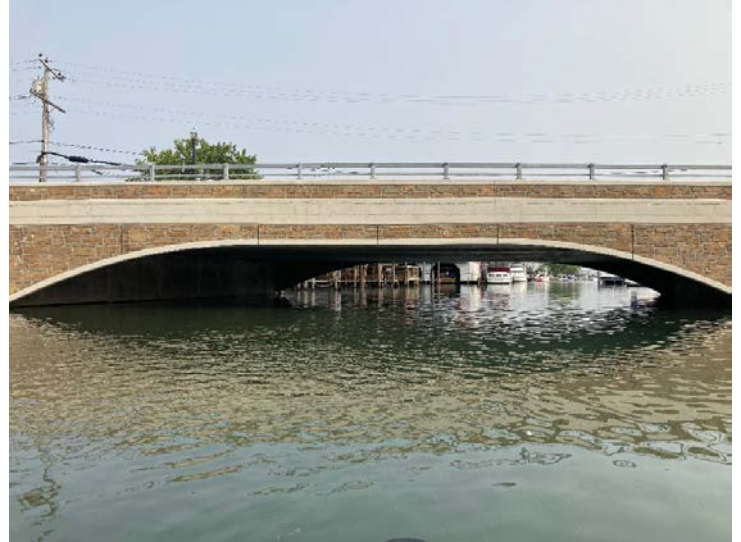
Document Name: IMG_4529.JPG Category: Elevation Span Number: Comments: South elevation
