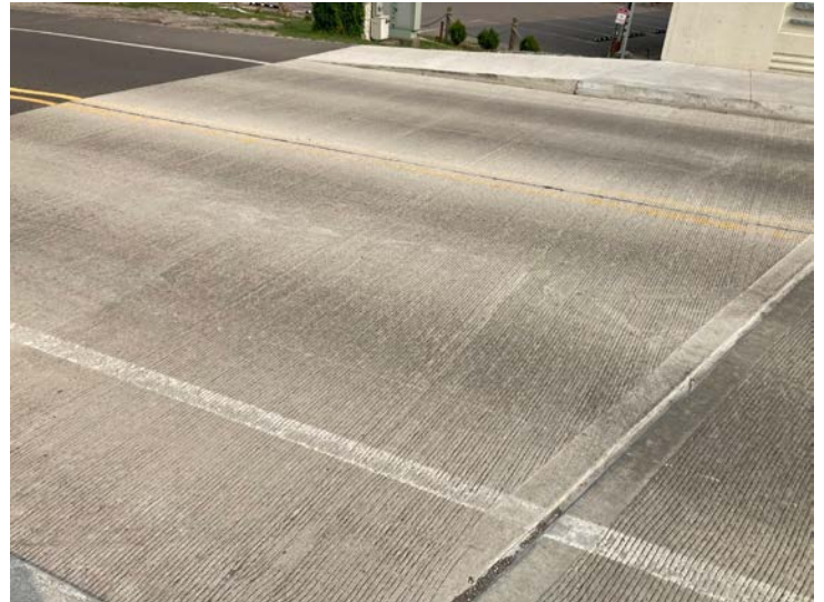
Document Name: IMG_4512.JPG Category: Approach Span Number: Comments: West approach
