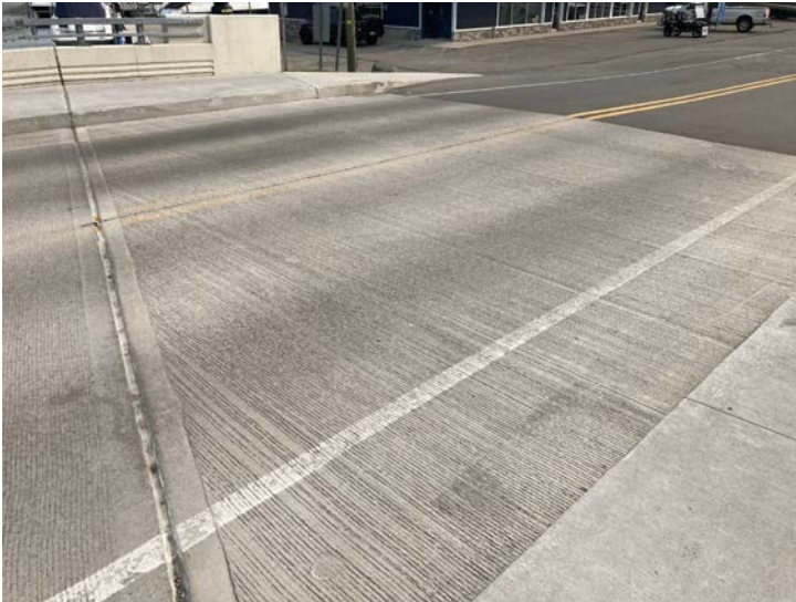
Document Name: IMG_4516.JPG Category: Approach Span Number: Comments: East approach
