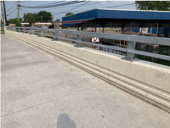
Document Name: IMG_4521.JPG Category: Railing Span Number: Comments: North rail
