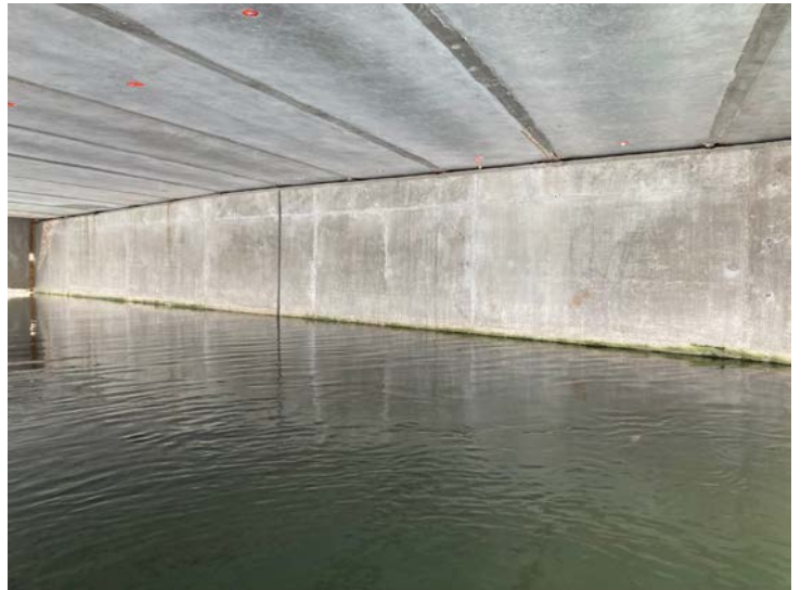
Document Name: IMG_4526.JPG Category: Substructure Span Number: Comments: West abutment
