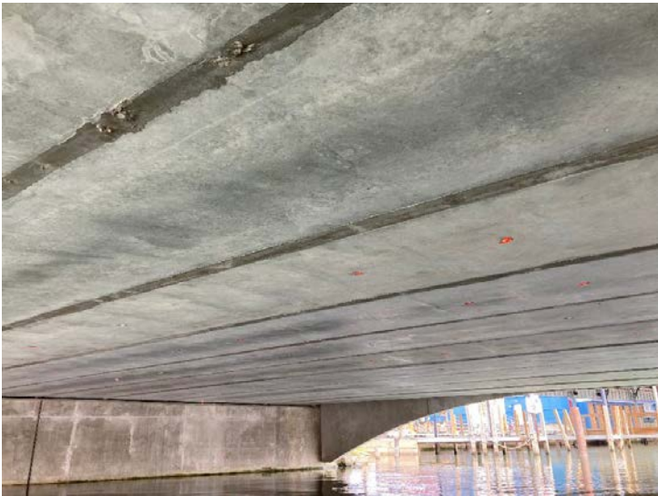
Document Name: IMG_4528.JPG Category: Superstructure Span Number: Comments: Beams
