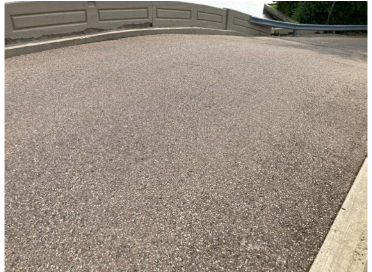
Document Name: IMG_4576.JPG Category: Deck Span Number: Comments: HMA surface
