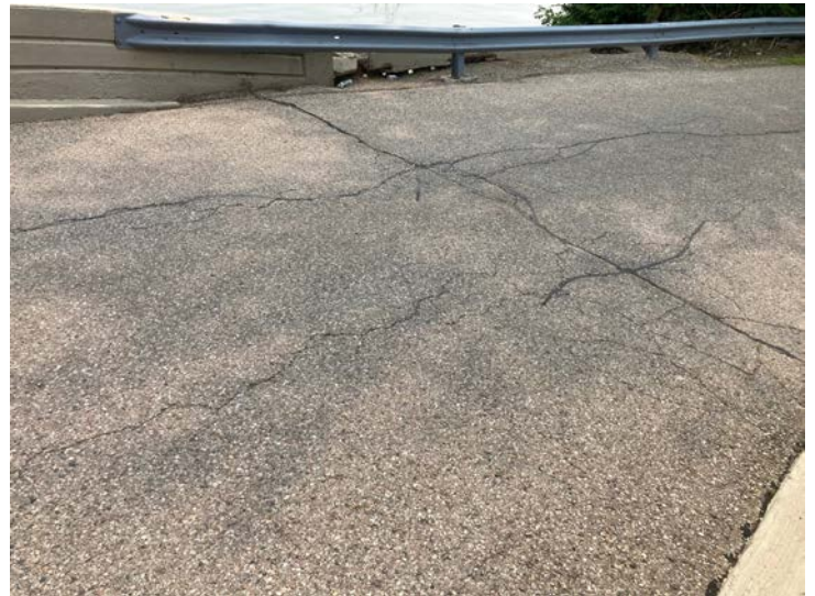
Document Name: IMG_4577.JPG Category: Approach Span Number: Comments: East approach
