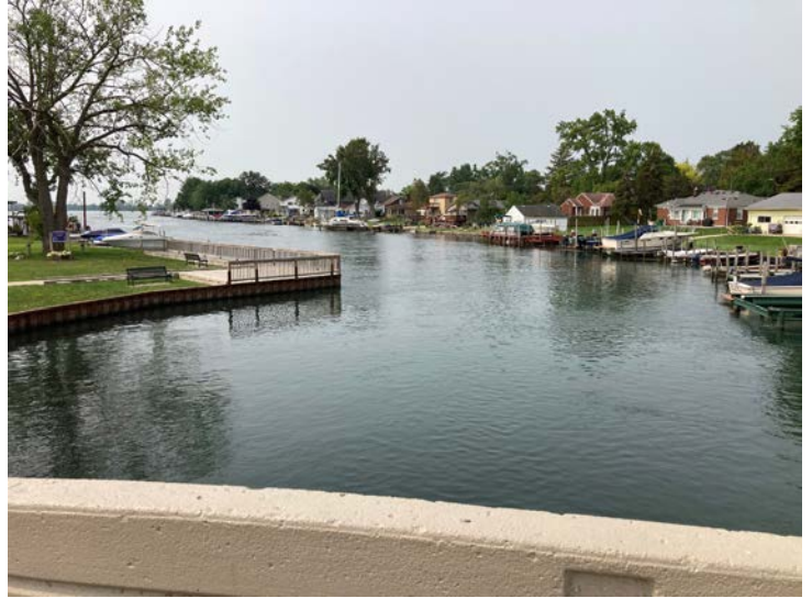
Document Name: IMG_4579.JPG Category: Channel Span Number: Comments: South channel
