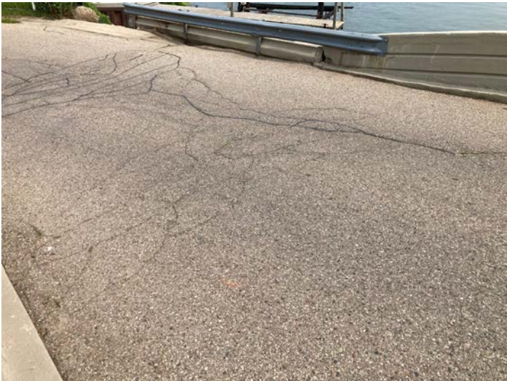
Document Name: IMG_4575.JPG Category: Approach Span Number: Comments: West approach
