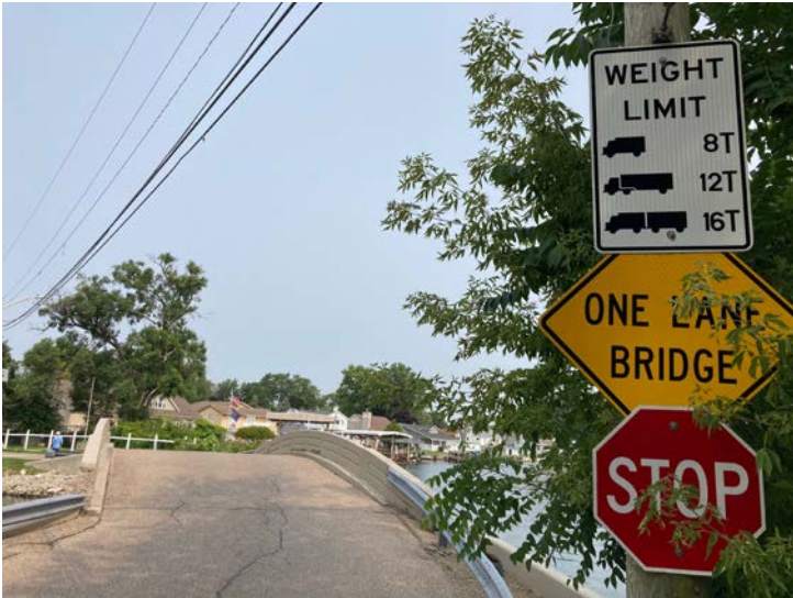
Document Name: IMG_4573.JPG Category: Posting Span Number: Comments: WB load posting
