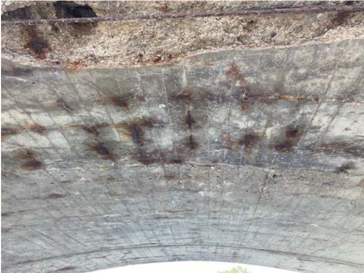
Document Name: IMG_4587.JPG Category: Superstructure Span Number: Comments: Top of arch
