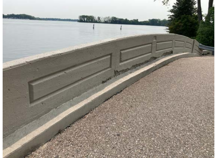
Document Name: IMG_4580.JPG Category: Railing Span Number: Comments: North rail
