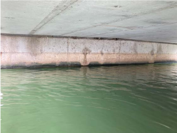
Document Name: IMG_4608.JPG Category: Substructure Span Number: Comments: Pier 1w
