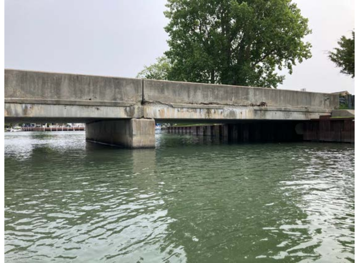
Document Name: IMG_4610.JPG Category: Elevation Span Number: Comments: South elevation
