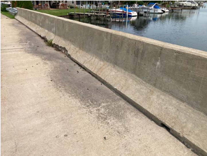
Document Name: IMG_4603.JPG Category: Railing Span Number: Comments: North rail
