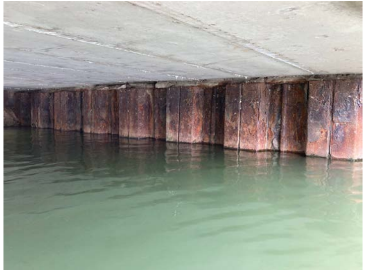
Document Name: IMG_4607.JPG Category: Substructure Span Number: Comments: West abutment
