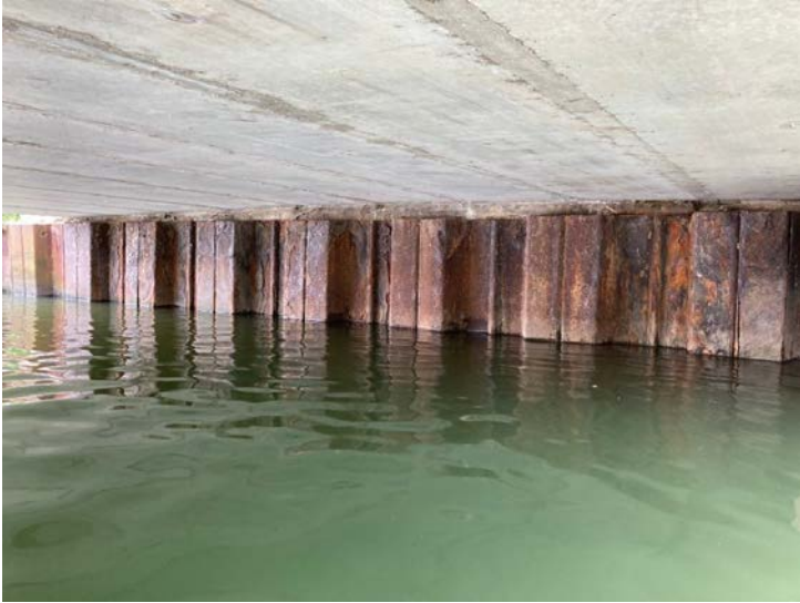
Document Name: IMG_4613.JPG Category: Substructure Span Number: Comments: East abutment
