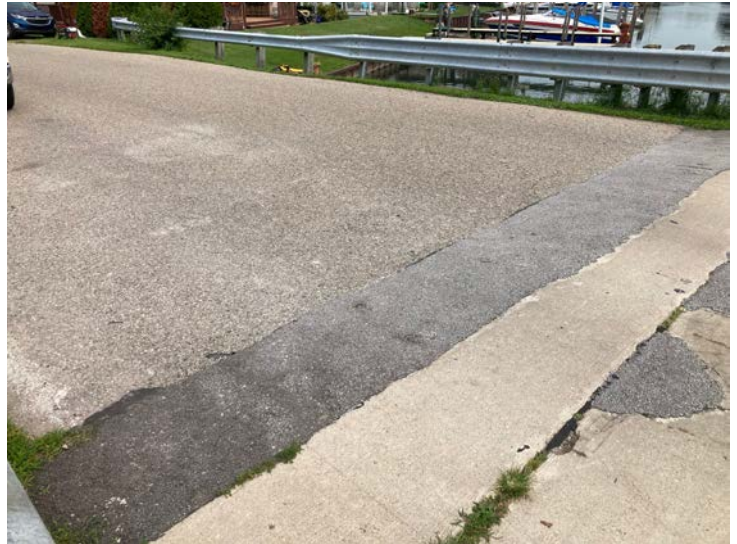
Document Name: IMG_4594.JPG Category: Approach Span Number: Comments: West approach
