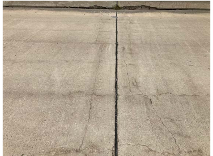
Document Name: IMG_4597.JPG Category: Joints Span Number: Comments: Joint 1w
