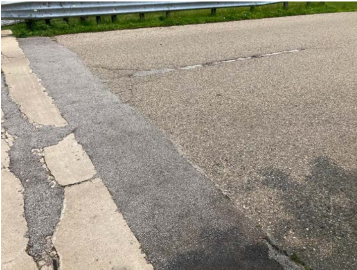
Document Name: IMG_4600.JPG Category: Approach Span Number: Comments: East approach
