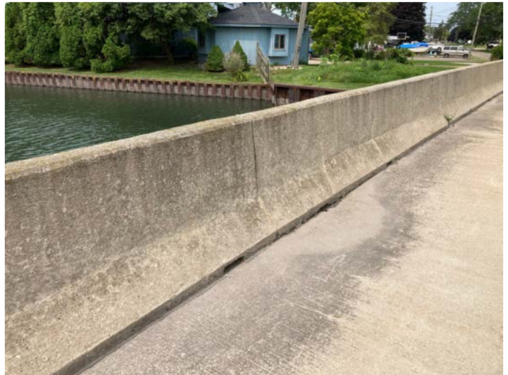
Document Name: IMG_4601.JPG Category: Railing Span Number: Comments: South rail
