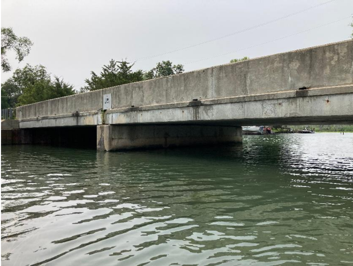
Document Name: IMG_4606.JPG Category: Elevation Span Number: Comments: North elevation
