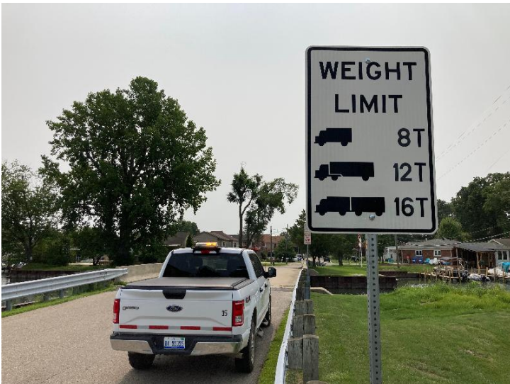
Document Name: IMG_4591.JPG Category: Posting Span Number: Comments: EB load posting
