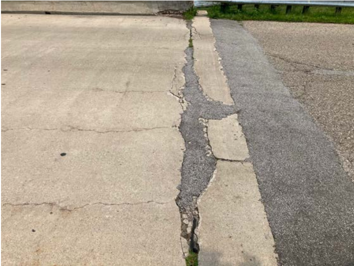
Document Name: IMG_4599.JPG Category: Joints Span Number: Comments: east reference line
